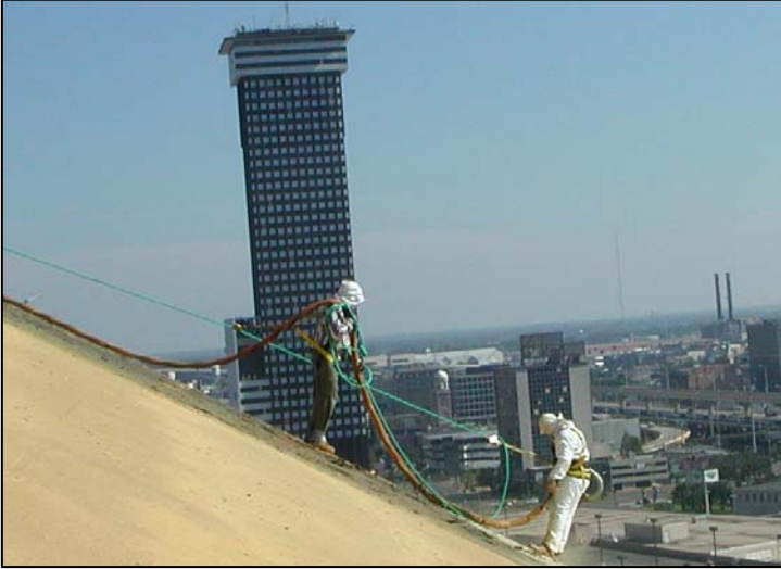
Spray Foam Roof Repair after Katrina (Louisiana Superdome)
